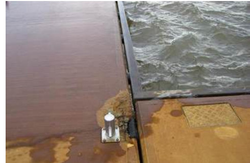
Figure 7: Floating house affected by micro organisms
